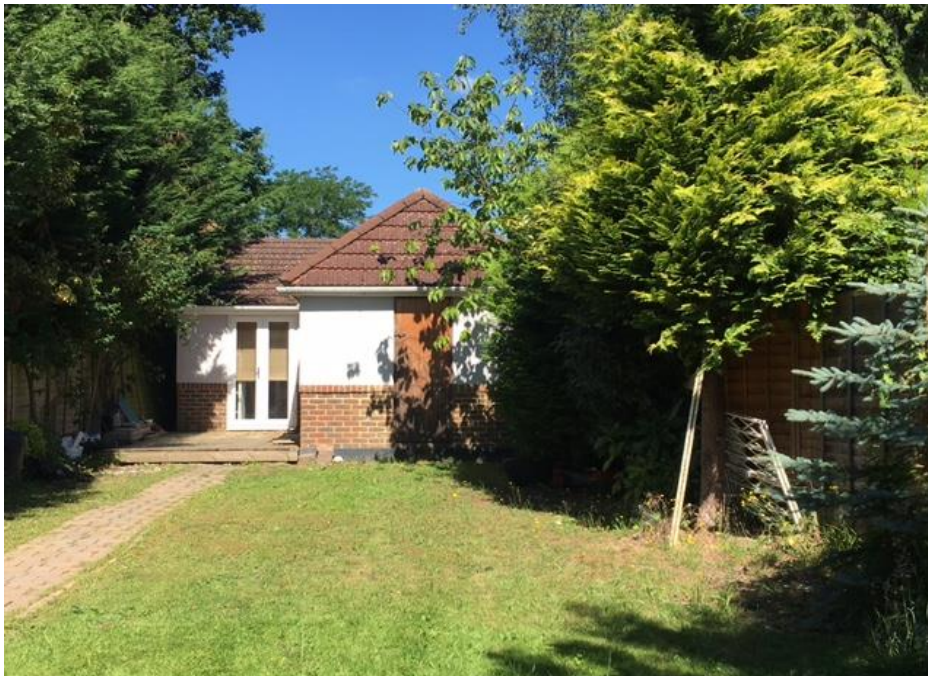
Rear garden of No.1 Wynlie Gardens
