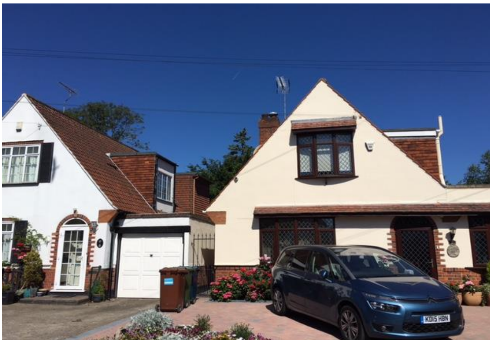
Photo showing front elevation of No.5 Wynlie Gardens (Left) and No.3 Wynlie Gardens (Right)
