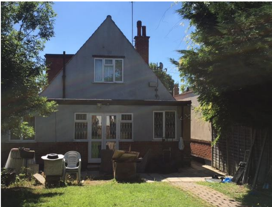
Rear elevation of No.1 Wynlie Gardens.
