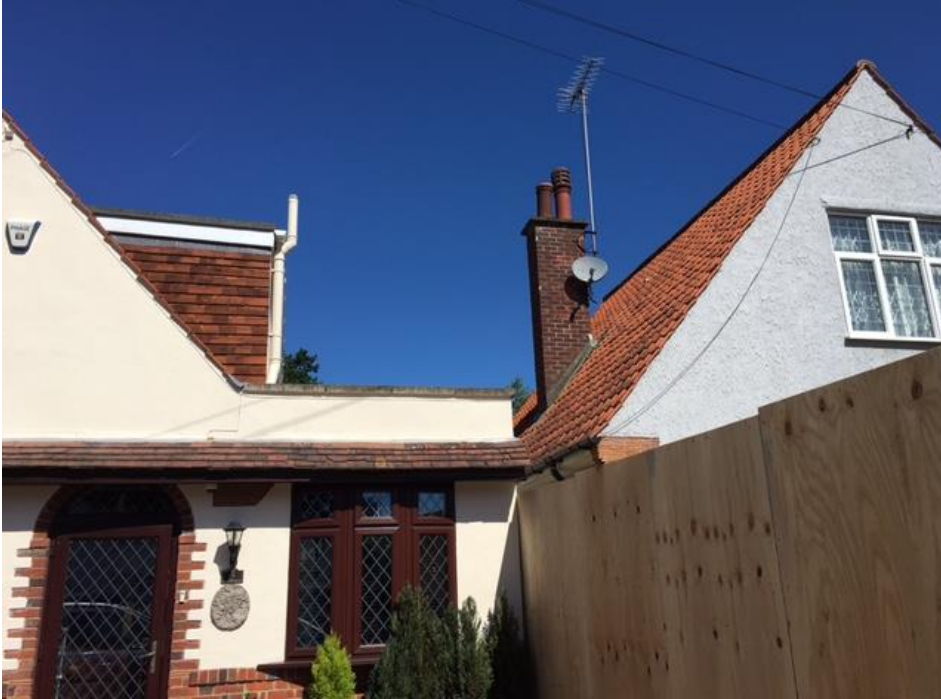
Photo showing the relationship between the front elevation of No.1 Wynlie Gardens (Right) and No.3 Wynlie Gardens (Left)
